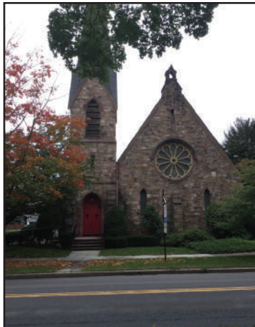
215 S Main Street St. James Episcopal Church CRGIS Key# 000614 NRHP Listed 11/20/1979
