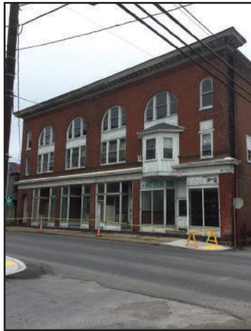
15 S Water Street Mozley's Opera House CRGIS Key# 155877
