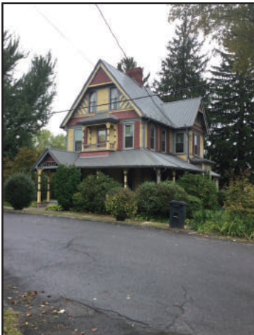
82 Kinsey Street Kinsey House CRGIS Key# 117939 SHPO Eligible 5/19/1990
